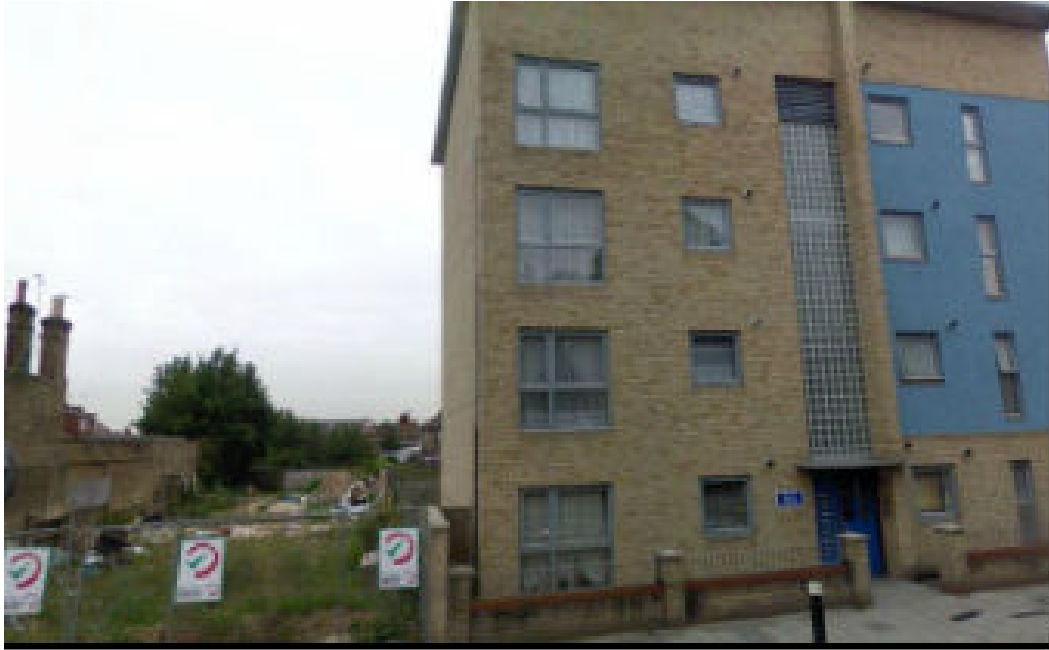
View from existing adjacent residential block
