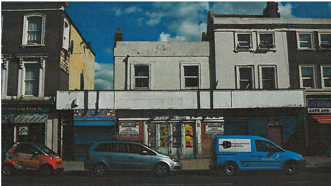
Existing Tottenham High Road Frontage
