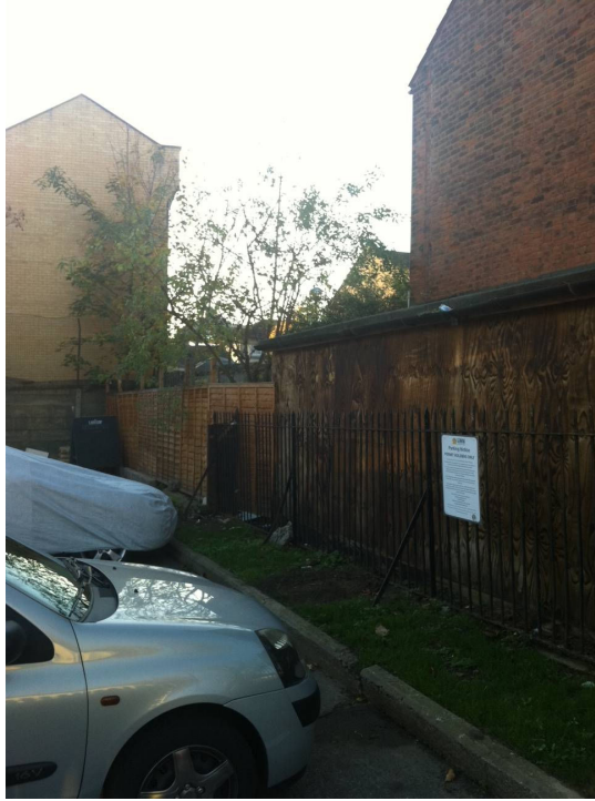
The 3 storey block at Khalsa Court, Acacia Road viewed from the carpark
